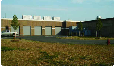
Above: The new power plant at the Brown Station Road Landfill Facility.
